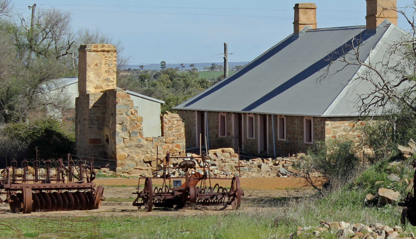
Image Credit: Macpherson Historical Homestead, one of the accommodation options offered to artists in residence. Photo courtesy of North Midlands Project.
